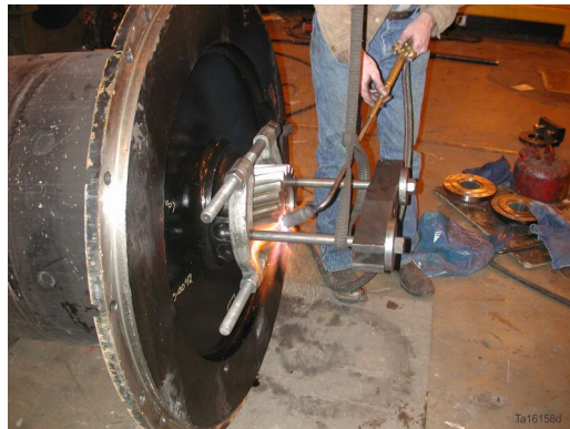
Figure 17. Heating the shell pinion
